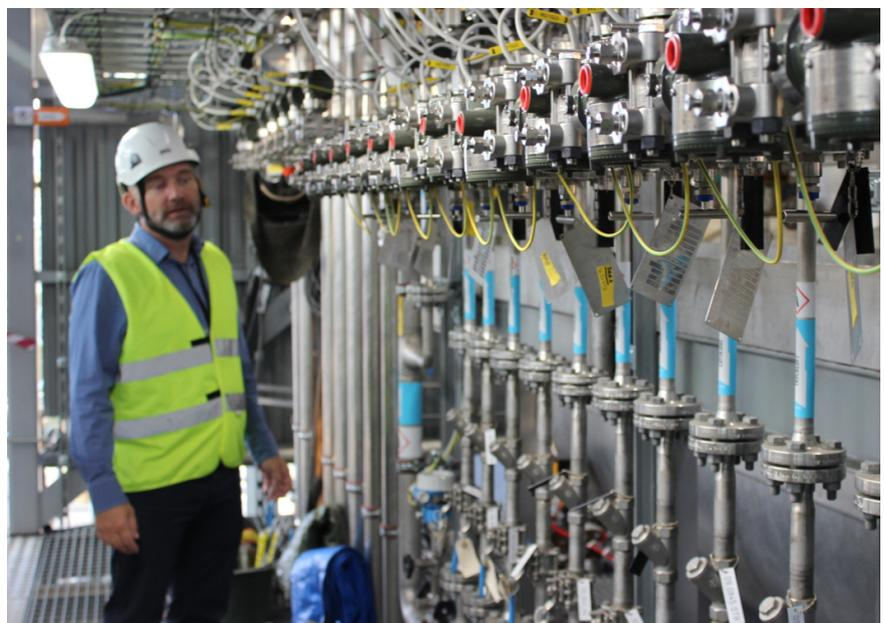
The gasification reactor has 14 infrared gas burners, each of which has its own piping and control systems.
